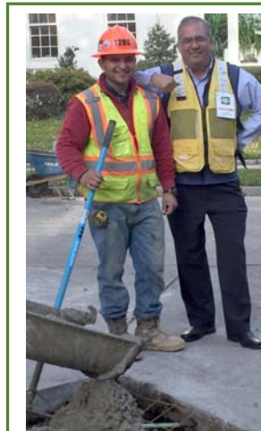
Mayor Riscica with workers pouring concrete on Plandome Court
