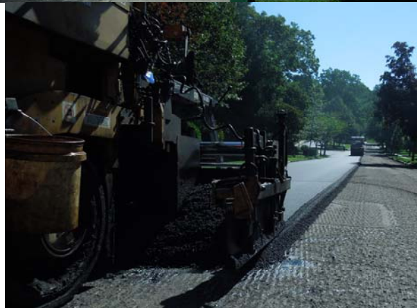
Town of North Hempstead contractors paving Webster Avenue in June 2015
