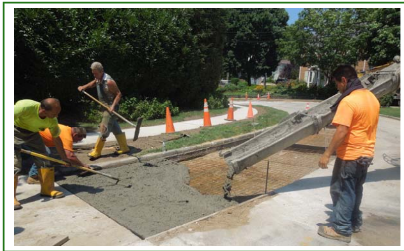
MLWD contractors restoring concrete road on Grandview Circle in Plandome Heights
