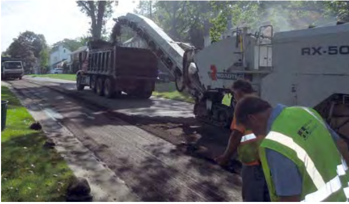
Milling on Cove Drive
