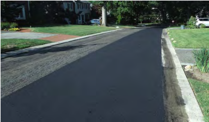
Paving on Cove Drive
