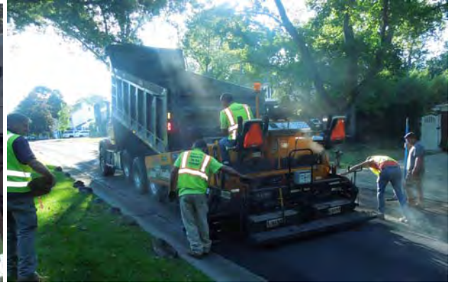
Paving on Cove Drive
