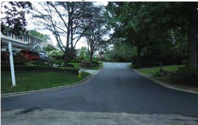
Paving on Willow Court
