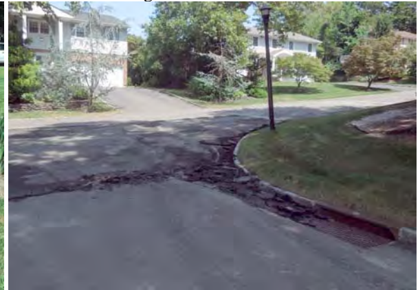
Repairs on Shore Road
