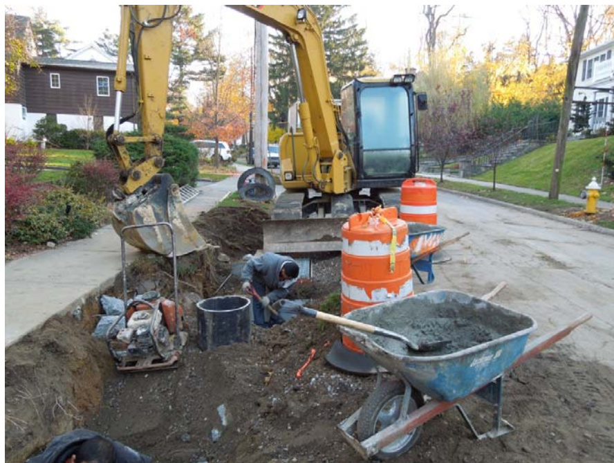
Storm drains being added to Bay Driveway in Plandome Heights
