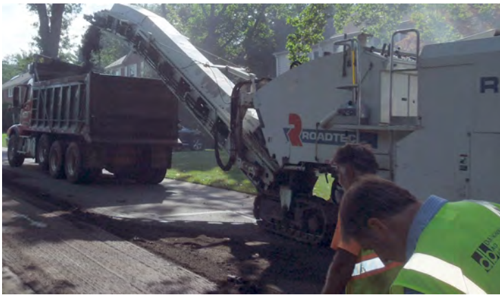
Milling operation on Cove Drive in 2018
