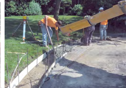
Swale/Gutter repairs
