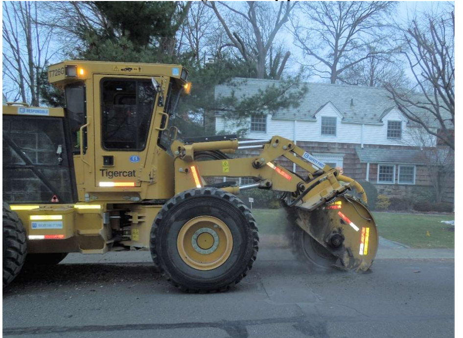
Breaking the pavement
