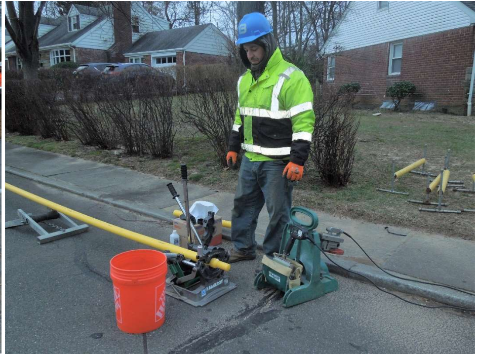
“Fusing” the PVC pipe
