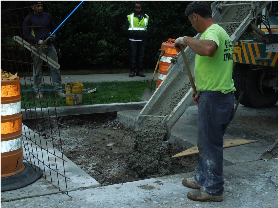
Concrete road repairs, 2018
