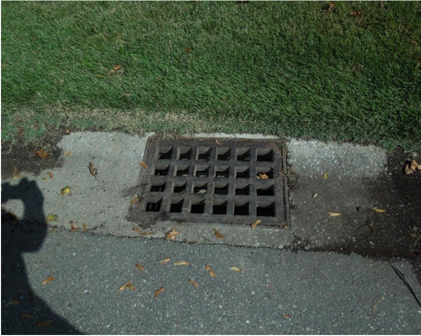
Existing storm drain - Waterway at Cove
