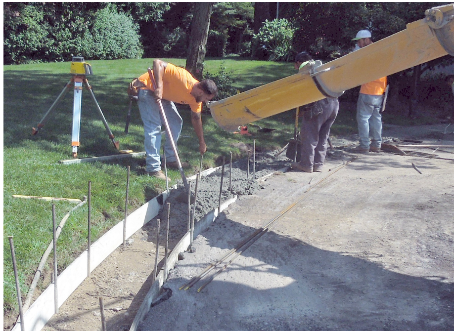
Swale and gutter repair, 2018
